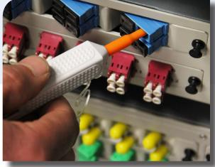
Fibre optic cleaning is one of the most basic, important and often overlooked procedures for maintaining fibre optic networks. FOS offers a comprehensive selection of Fibre optic cleaning & consumables for your factory or on-site termination and maintenance needs. FOS supplies a complete range of one-click cleaners, cartridge cleaners, cleaning sticks, lint free wipes and other cleaning products.
