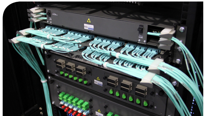
Individual sliding trays for each row of cassettes allow for simple patching, cassette insertion and removal and unparallelled finger access
